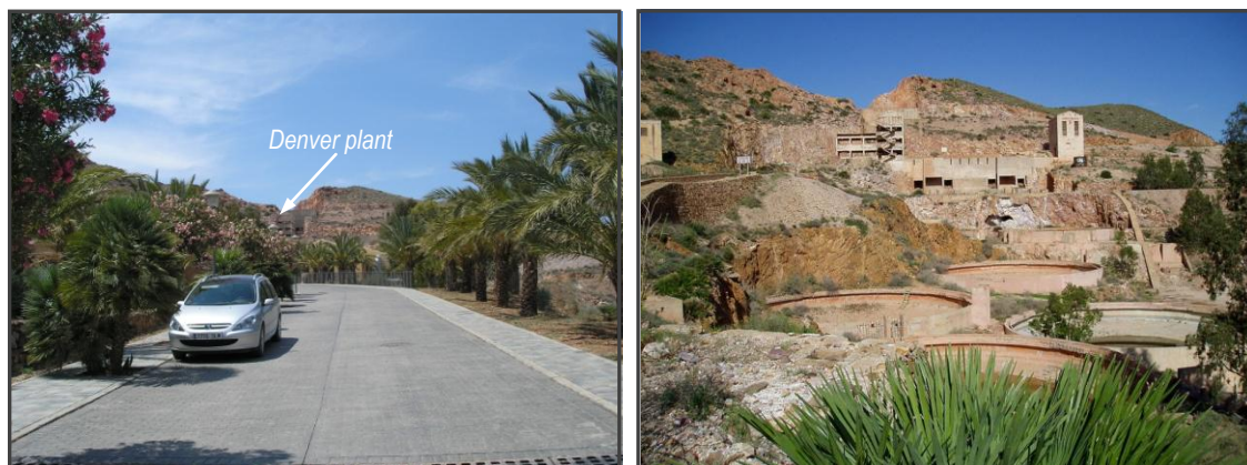
Left, the initially cobbled road that goes from Rodalquilar to Los Albaricoques (the car is in the opposite direction); in the background: the Denver Plant. Right, the Denver gold ore hydrometallurgical plant; in the foreground the cyanidation tanks (vats); above the ore milling plant (Wikinauta 2008).
